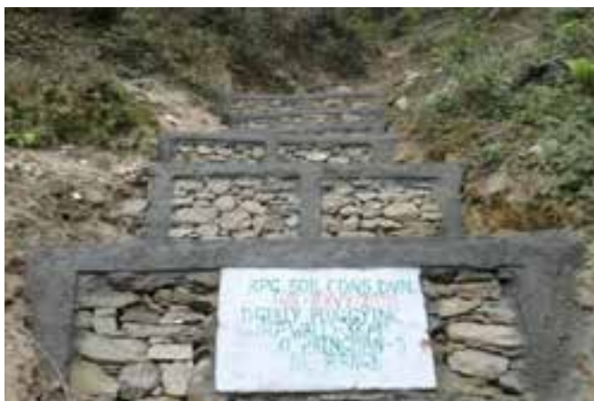
Gully plugging at Paingoan -9 under Relli Catchment Range (RKVY)
