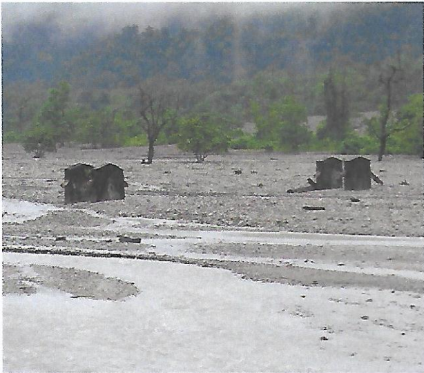
Huge deposit of boulders and debris on Jainty river. The bridge on left is covered with debris accumulated over the years.
